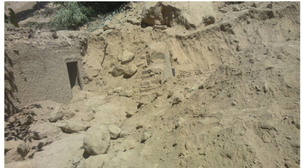
Houses destroyed by landslide in Takhar, Chah Ab District, Zaker Abad village Photo Credit: CONCERN Worldwide
