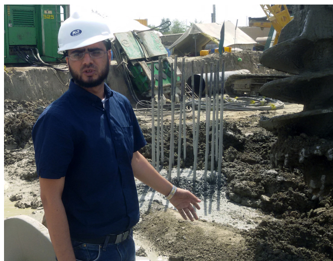
A TRQN participant supervising a construction project in Kabul
